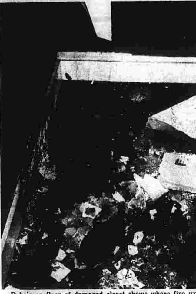
Debris from a damaged apartment building shows where fire was started in the Centennial Apartments, Chestnut Street, Wednesday afternoon. Officials said the fire, similar to one at the same place on April 29, was "definitely set." Police are investigating. (Herald photo by Pinto)
